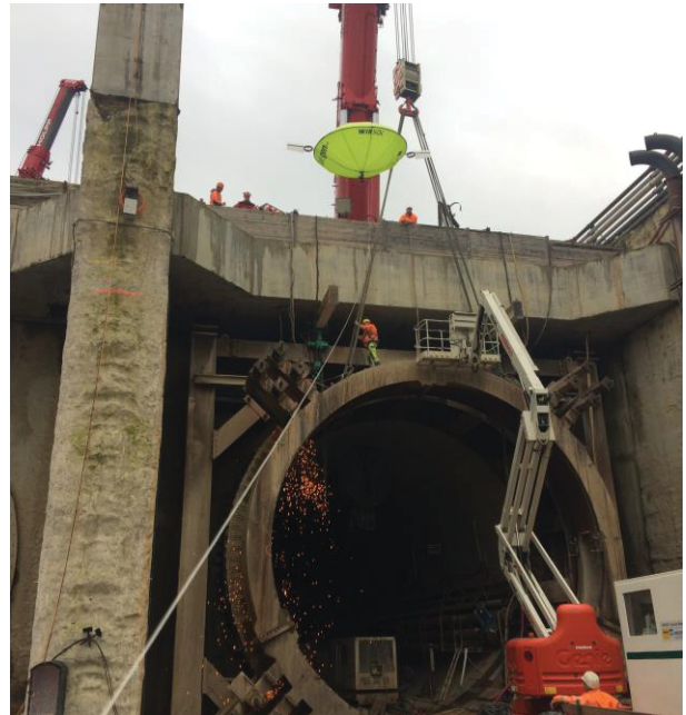
Image 6 Outdoor Tunnel Inspection (a.I)
