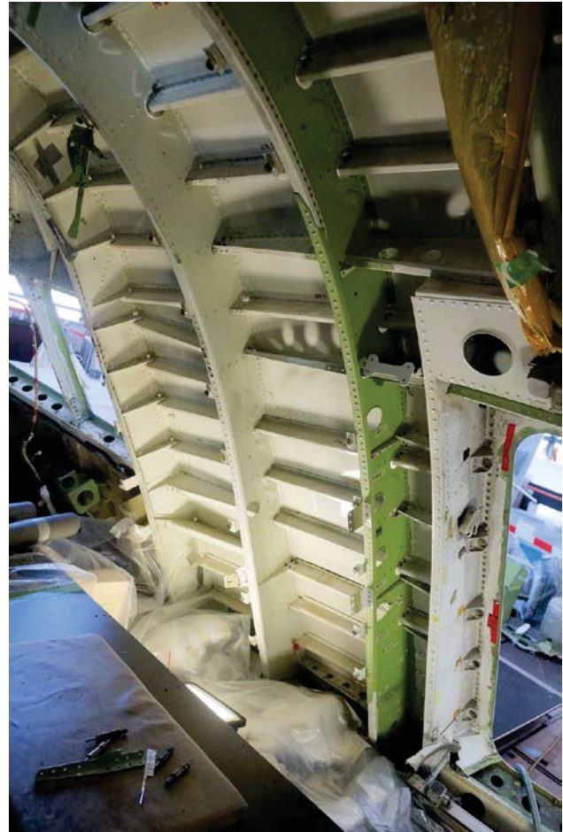
Bild 11. New Frame RH380 (green) installed.
